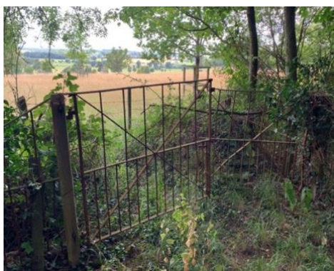
Small park gates
