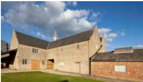
Coleshill's new Heritage & Skills Centre
